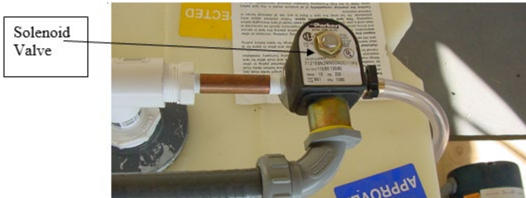
Figure 3: Normally closed solenoid valve
