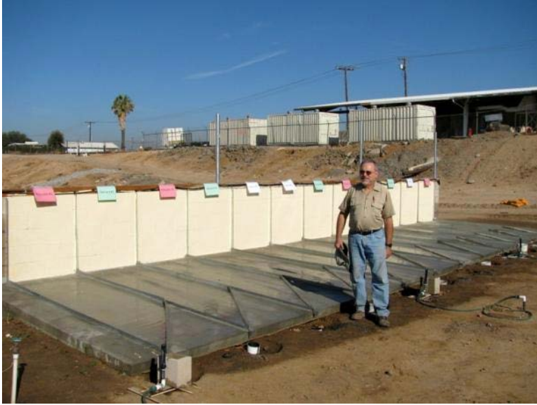
Figure 1. One side of constructed wall showing 12 3-ft wide segments.
