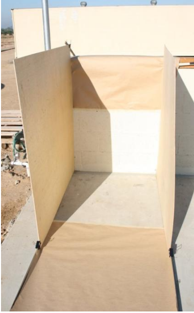
Figure 3. Masking an area to be treated.
